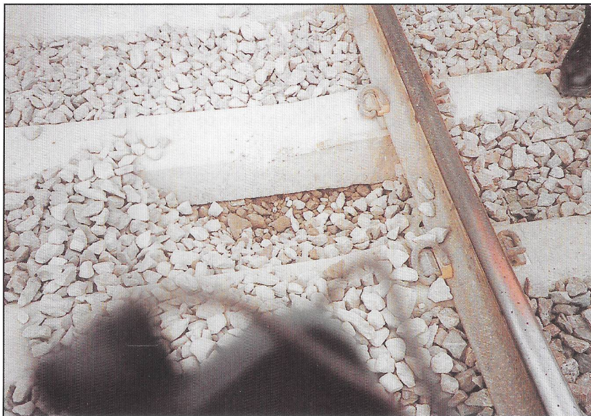
Done in a Fashion ... Ballast pyramid not excavated!
