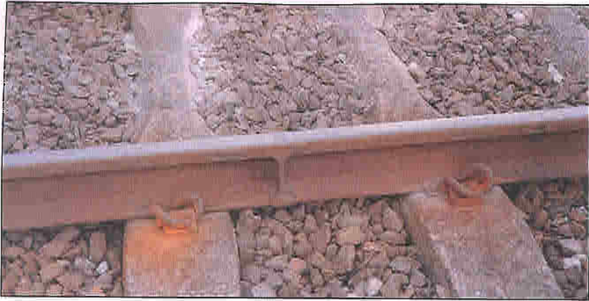
Pads out on a weld. Onset of a wet bed.
