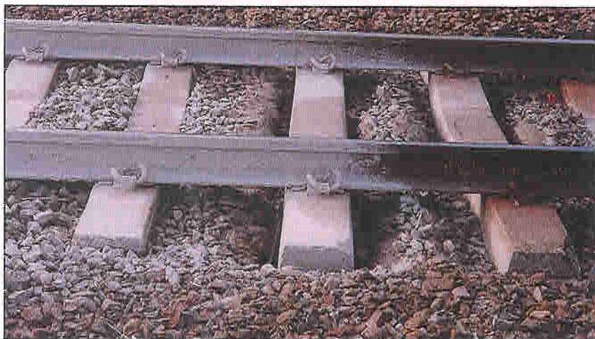
Voids: Water under pressure washes out ballast
