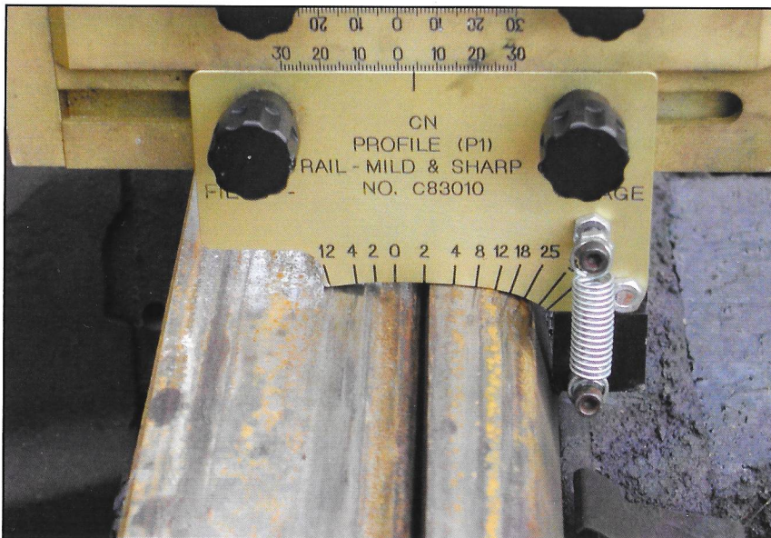
Template on Closed Switch (Un-ground)
