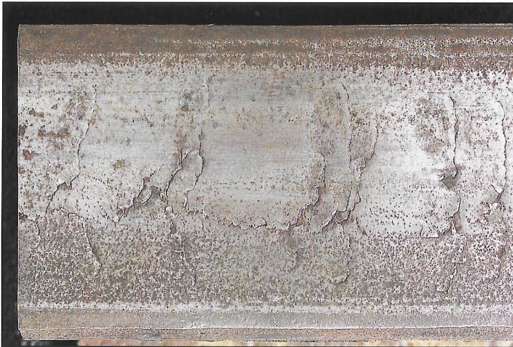
False Flange Damage
