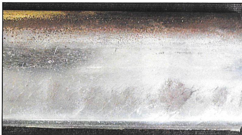
Head Check Cracks with "Shadows"
