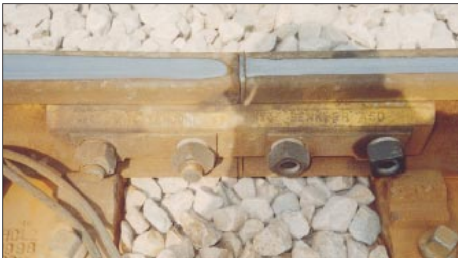
Figure 7 Benkler 4 Hole Nylon Encapsulated Joint.
