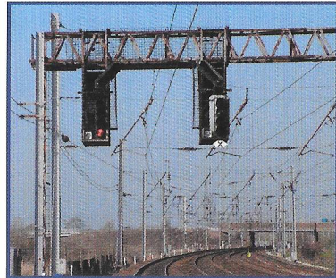
Four aspect signal capable of showing a red or 2 yellows or a green light *Note the positioning of these signals on a gantry
