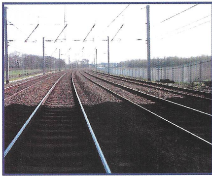
Four Track Situation Consisting of: Up Fast Line Down Fast Line Up Slow Line Down Slow Line
