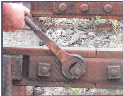
Secondly a small spanner can be used to ease the fishplate off (not fully) to a position where the lubricant can be applied behind the plate.
