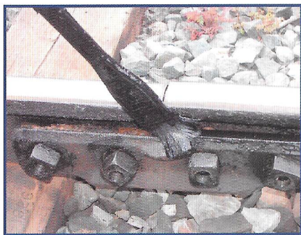
Now the lubricant can be applied with a long handled brush, this type of brush allows the worker to get right inside the rear of the fishplate keeping fingers clear a all times.
