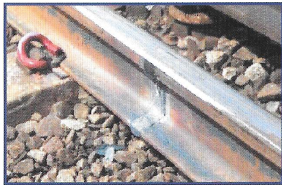
Stage 4 Grinding and profiling of the rail
