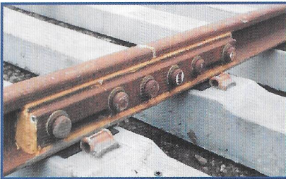
A manufactured six hole insulated (glued) joint
