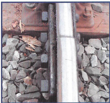
Firstly the bolts are eased off with a long handled fishbolt spanner.
