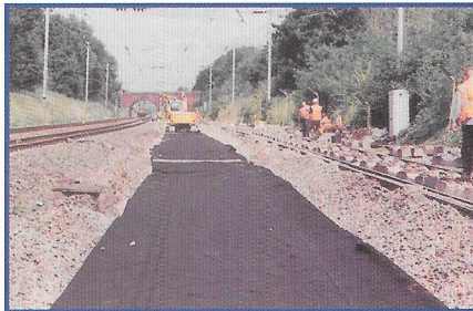
Installation of Subgrade layer
