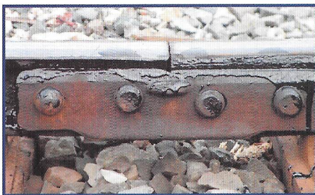
Lastly the fishplate bolts are run back up to the correct torque, the diagram illustrates the finished product.
