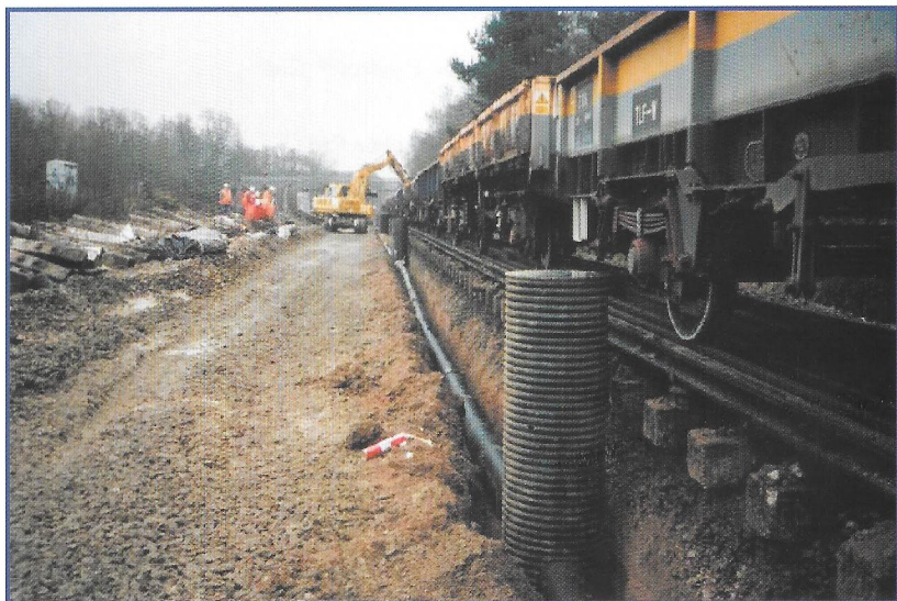
Above we see the digging out and positioning of a new six foot drain and catch-pits. The catch-pits are cut down to size later.
