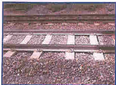
The result of neglected drainage, advanced stages of ballast attrition.
