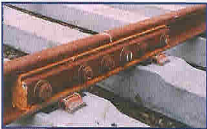
A manufactured six hole insulated (glued) joint
