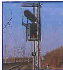
A three aspect signal with route indicator to indicate when trains are to transfer from one line to another
