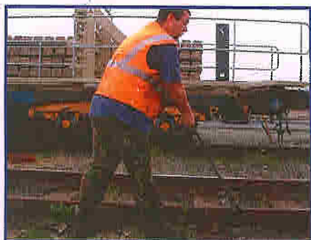
Firstly the bolts are eased off with a long handled fishbolt spanner.
