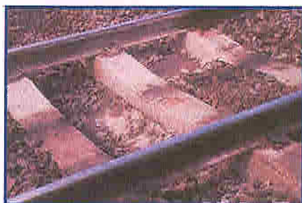
The result of neglected drainage, advanced stages of ballast attrition.
