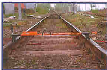
Cross-Level Readings are Taken
