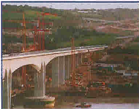
A major item of work, the construction of a new rail bridge
