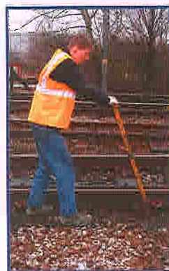
Panpuller / Extractor used for inserting and extracting Pandrol™ clips
