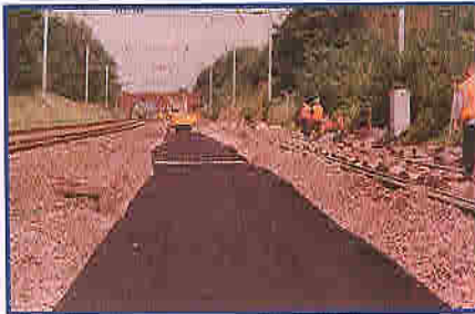
Installation of Subgrade layer
