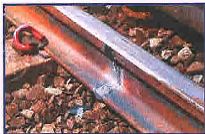
Stage 4 Grinding and profiling of the rail
