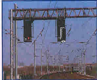
Four aspect signal capable of showing a red or 2 yellows or a green light
