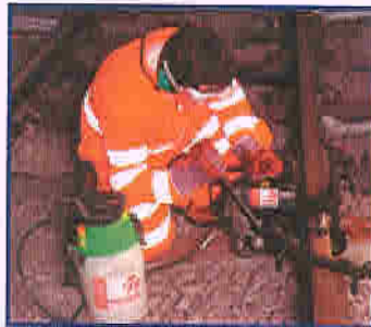
Cembre Rail Drill for drilling rails
