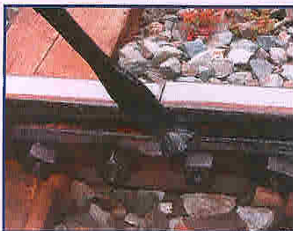
Now the lubricant can be applied with a long handled brush, this type of brush allows the worker to get right inside the rear of the fishplate keeping fingers clear at all times.
