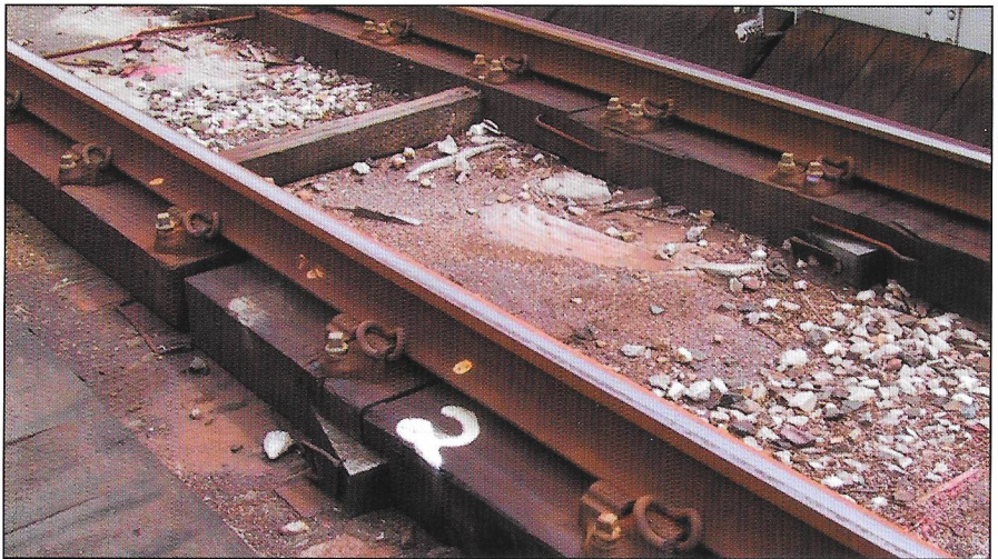
Figure 6 Although there is no laid down minimum length for a longitudinal timber they should be as long as the track design allows. Short timber lengths are bad practice which should be avoided.
