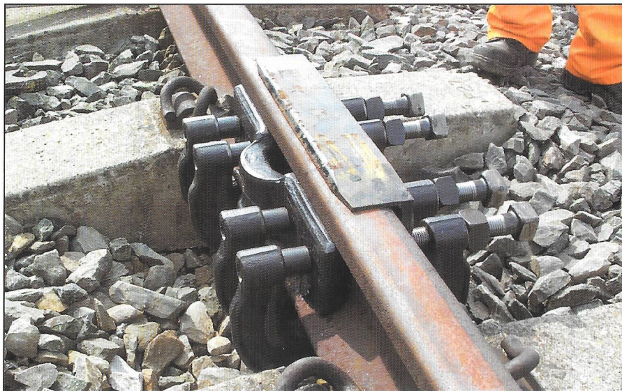
Fig 10. An emergency bridging piece
