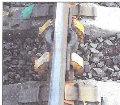
Clamps fitted correctly to both rails prior to tightening
