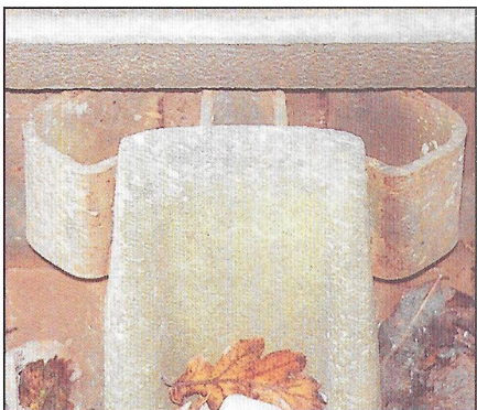
Correctly positioned Panlock Key
