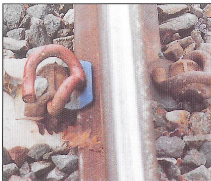
Examples of a correctly installed Bullhead rail fastening (left hand photo) Flat Bottom rail fastening. (right hand photo)
