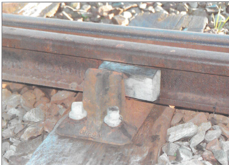
A correctly installed wooden Bullhead key
