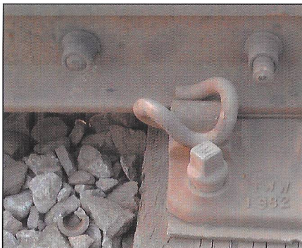
The incorrect use of rail fastenings
