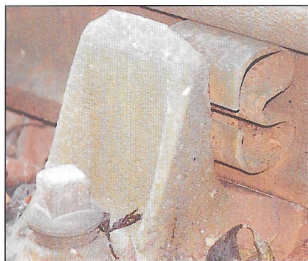
Examples of a correctly installed Bullhead rail fastening (left hand photo) Flat Bottom rail fastening. (right hand photo)
