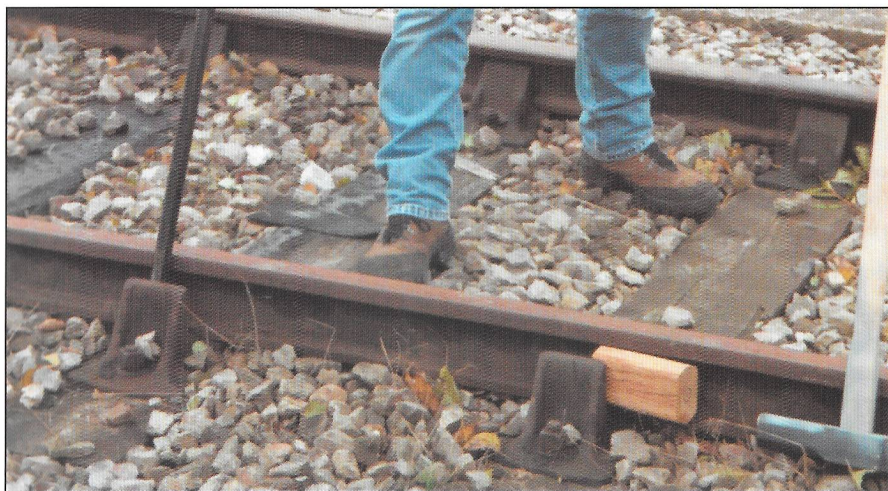
The use of a rail bar to correctly position the rail in the jaw of the chair
