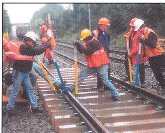
Staff using FASTCLIP installation equipment in a five man team
