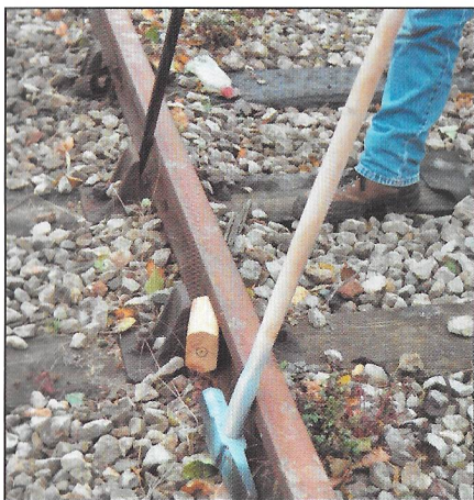
Initial placing of the key prior to striking
