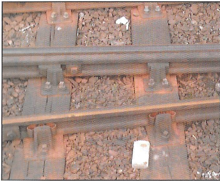
The correct use of rail fastenings
