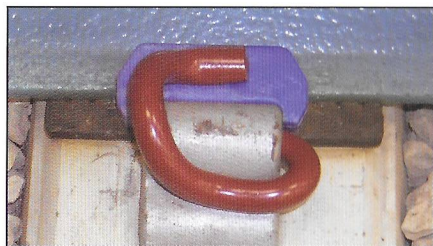
Clip Fastening assembly as used on the F40 Sleeper
