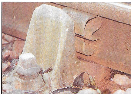
A correctly installed Tapered Steel Bullhead Key
