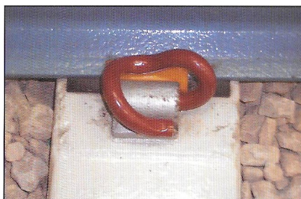
Pandrol PR Assembly for F27 Sleeper
