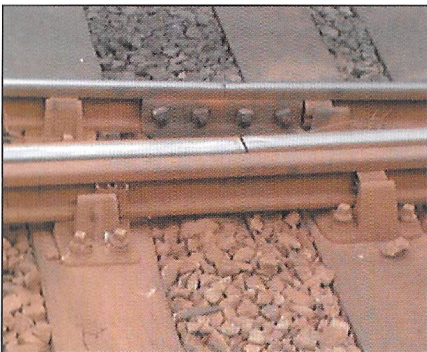
The incorrect use of rail fastenings
