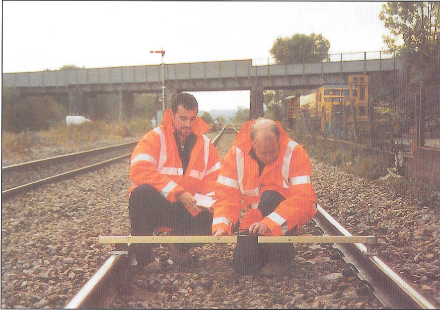
Photograph - measuring cross-level
