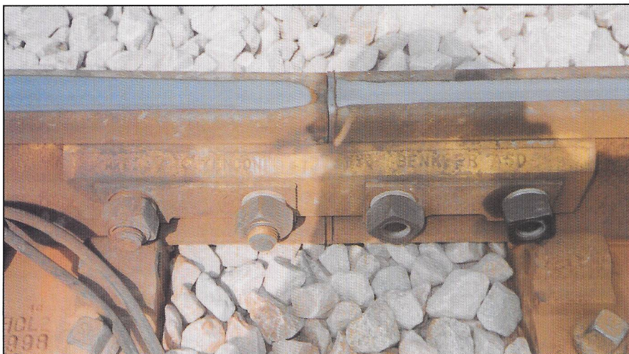
Figure 7 Benkler 4 Hole Nylon Encapsulated Joint.
