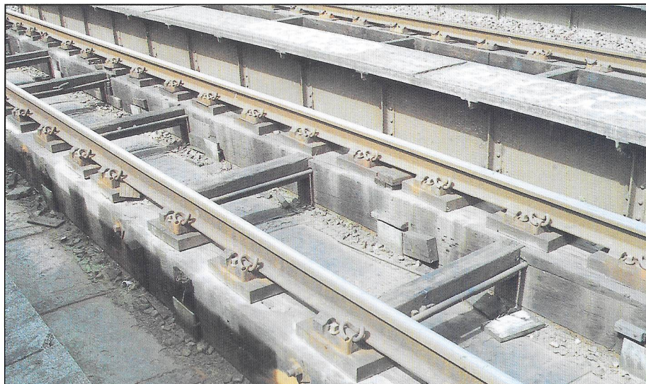
Figure 11 Longitudinal timbers require detailed attention
