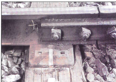
This fishplate has crept so much that the elastic spike has been reversed and only holds the baseplate in position. The baseplate is shuffling badly. The vee gap at the rail foot suggests that a sett has been used to adjust the rails.
