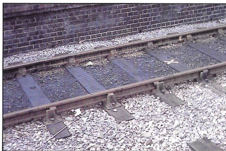
Keys correctly driven in alternative directions
